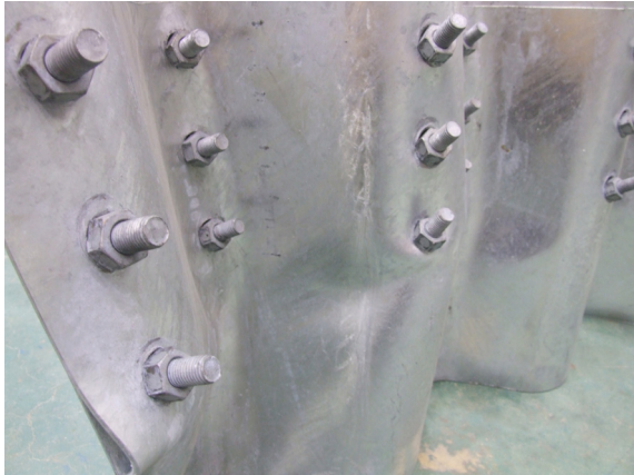
(a) combined failure with plate bearing and local buckling (I)
