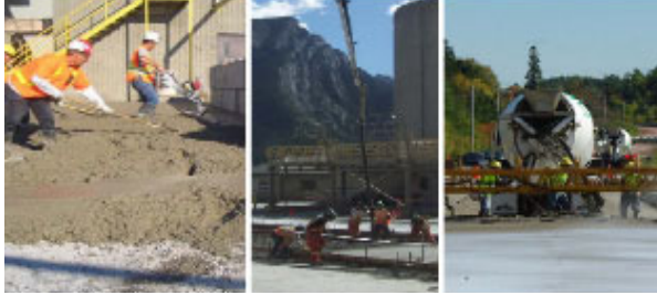
Fig. 3 Pavement Construction using LSP(Canada)
