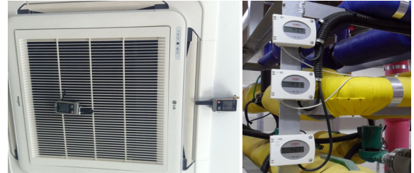
Fig. 4 Install measuring instruments.
