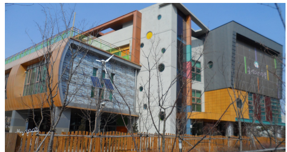
Fig. 2 Substantiation building whole view.
