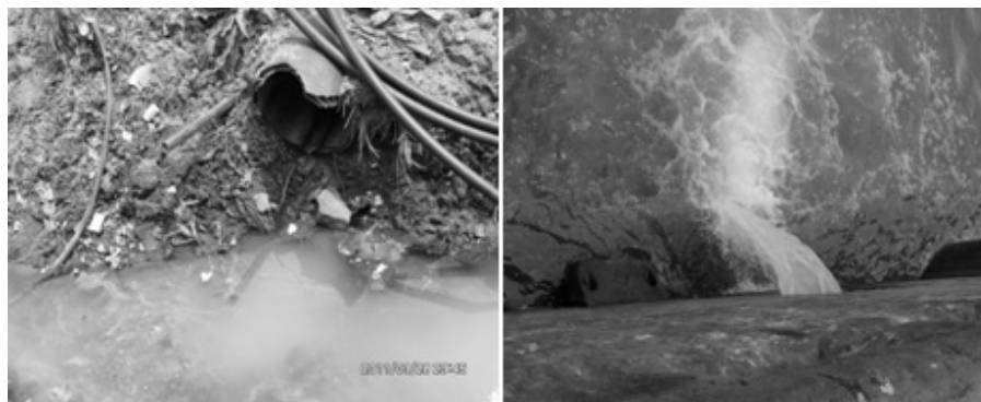
Fig. 2. Rainfall runoff discharge conduit to the shoreline
