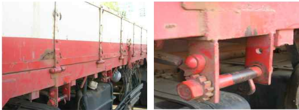
Figure 1. Fixation blocks welded to a truck
