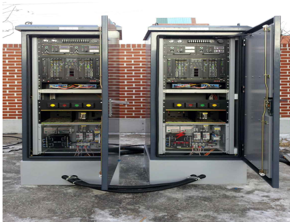
[Fig. 8] Installation of Up direction 3, 4 Site Output Unit
