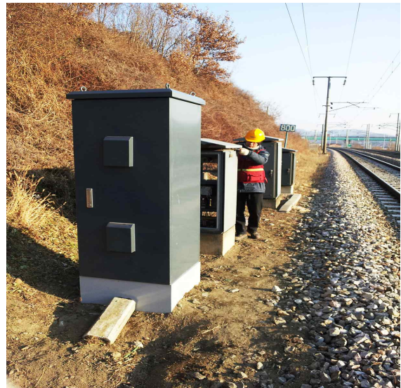
[Fig. 7] Installation of Up direction 2 Site Output Unit
