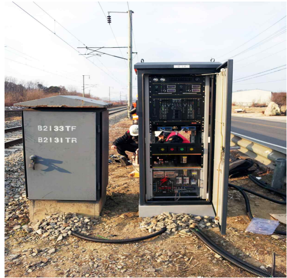
[Fig. 6] Installation of Up direction 1 Site Output Unit
