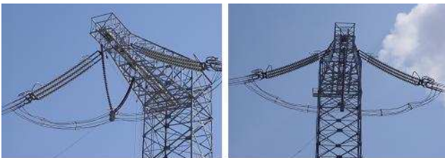
Fig. 2. Installation of the 765kV jumper V-string
