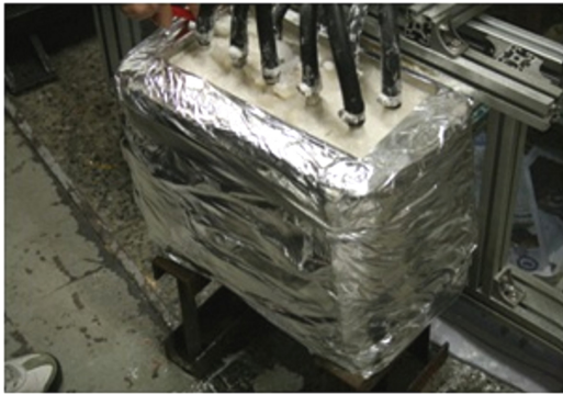
Photo. 3 Photograph of heat accumulator
