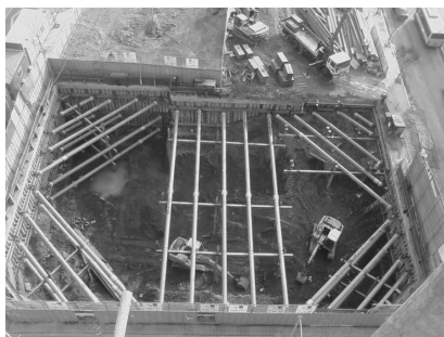
(a) Conventional strut system
