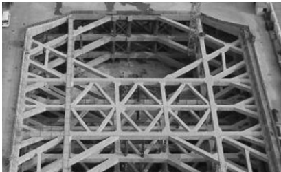
(c) CTS (Concrete Truss System)
