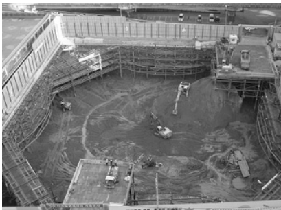
(b) IPS (Innovative Prestressed Support) system
