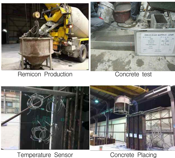
Temperature Sensor Concrete Placing Figure 2. CFT specimen for Fire resistance test
