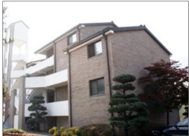
Fig. 1 Building installed the residential GSHP.
