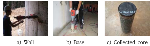
Fig. 8 Collect concrete core from base slab & wall
