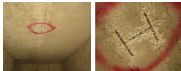
Fig. 11 Result of Water ponding test at H-Beam area
