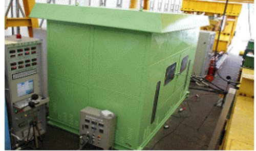
Figure 4: Feature of shield chamber surrounded by steel plates
