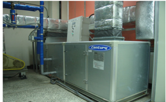
[Fig. 3] Experimental apparatus of central cooling system.
