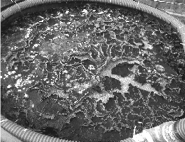
Fig. 6. Dry flake of algae formed from sludge cake on the surface of filter sand.
