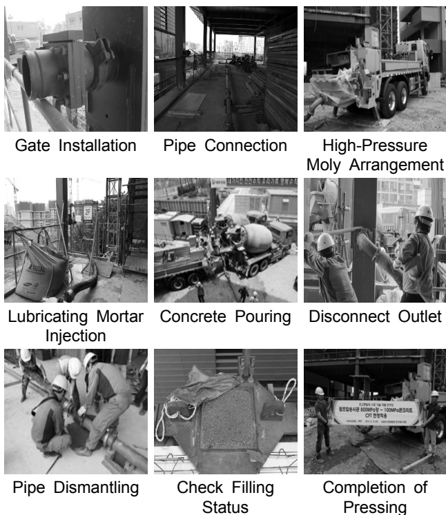
Fig. 5 Pressing Construction Processes
