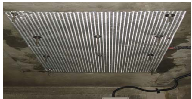
(c) Installation of anode
