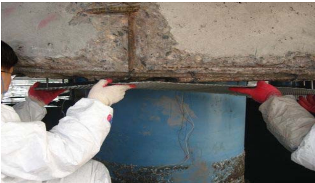
(c) Installation of anode
