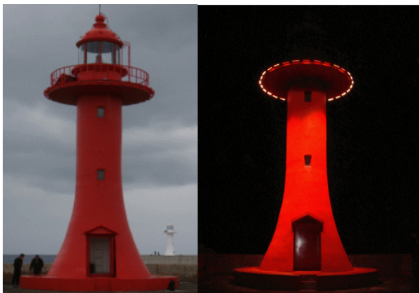
Figure 11: Pictures of breakwater lighthouse installing LED floodlight (Seogwipoochang in Jeju Island).
