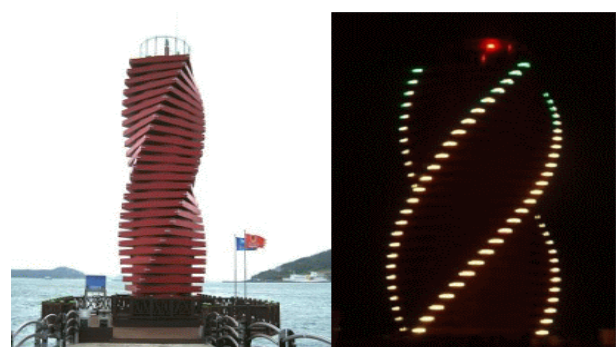
Figure 1: Wando Hang Lighthouse - Direct illumination Using the same color of illumination lighting and the A to N lighting can enhance conspicuity of A to N. It has helped mariners on the sea
