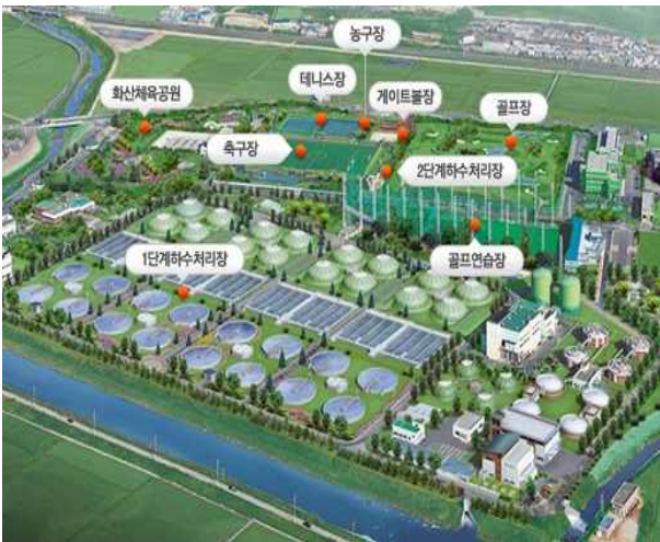
사진 1. ○○하수처리장 Photo 1. ○○Sewage treatment plant
