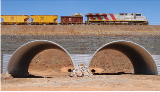
Fig. 2 Buried corrugated steel structures subjected to train
