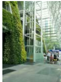
(a) Building A
