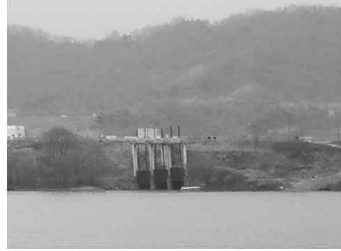
(b) After 4 river project (NakDong river, 2013)
