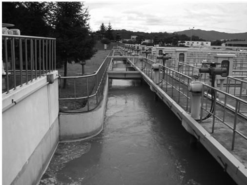
(a) Distribution open channel
