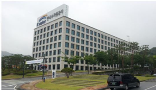
Fig. 1 External view of the building.
