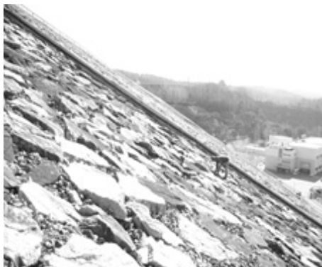
(a) The slope of rockfill zone
