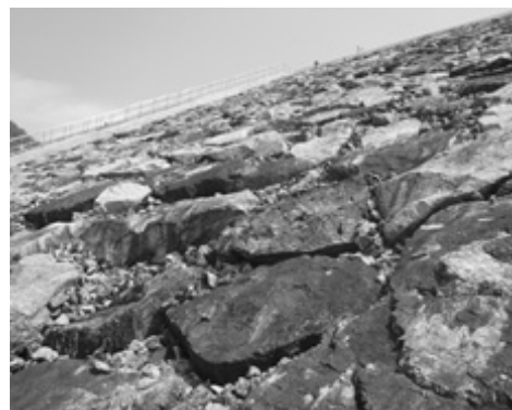
(b) Surface of rockfill zone
