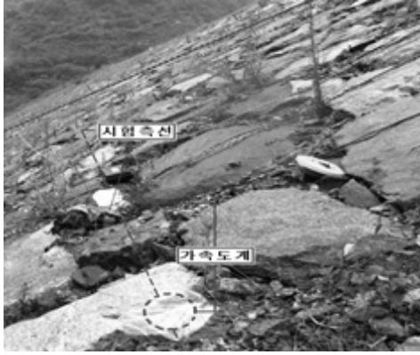
Fig. 12. HAWW test on the slope of the dam
