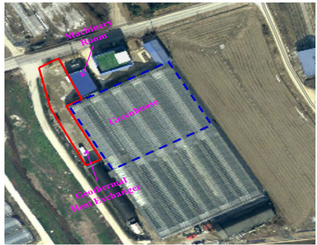
Figure 2. The aerial photo of the greenhouse.
