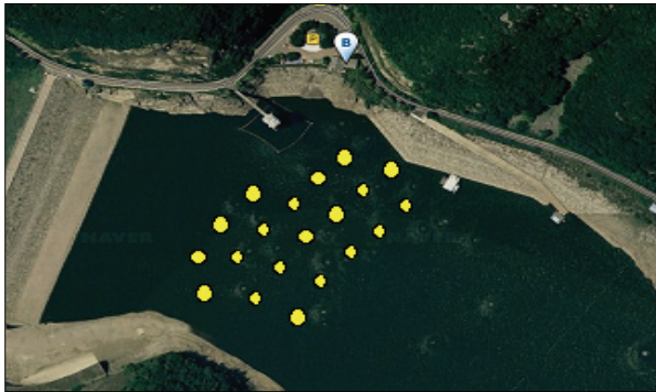
Fig. 8 Installation of water aeration
