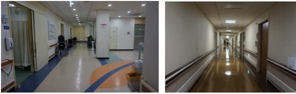
[Figure 5] Although the color, texture, handrail etc are considered, still corridors are functionally planned.
