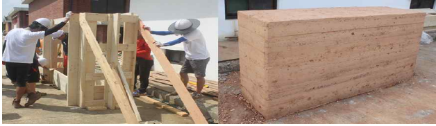
Figure 1. Rammed earth method(3)
