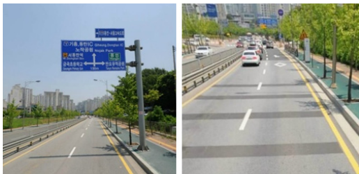
[Fig. 10] Access Traffic Road to New-town
