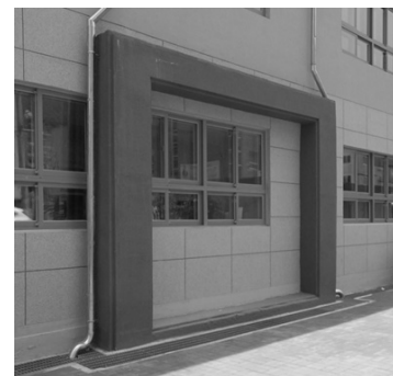
Fig. 3 R/C building strengthened with SRCF external connection method
