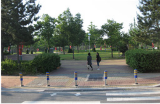
Fig. 1 Bollards installed along a road
