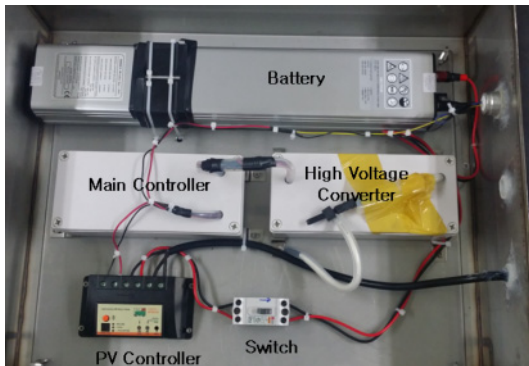
Fig. 3 Installation of water quality improvement system
