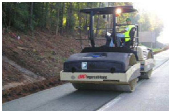
Fig. 1 Roller Compacted Concrete Pavement Method
