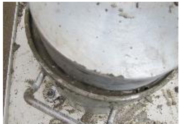
(b) Appearance of Mortar
