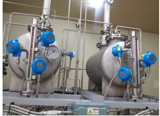
Fig. 6 Decanter of Hydrogen and Oxygen gas collection
