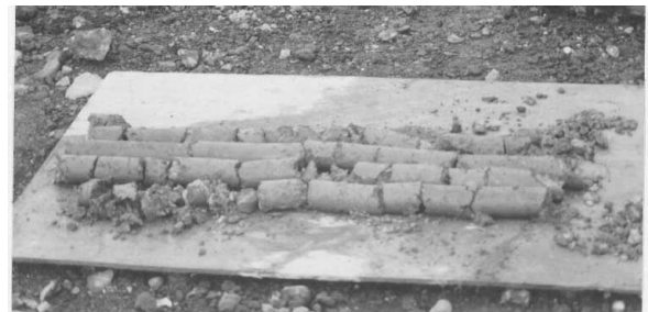
Fig. 7. Core sampling of the first test construction
