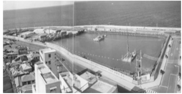
Fig. 4. The view during construction
