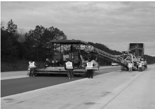
(a) Resurfacing of RCCP
