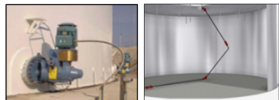
Fig. 1 Floating Roof Tank & Mixer
