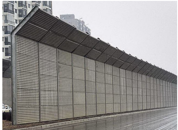
Fig. 4 Slanting the Top (Noise Barrier)
