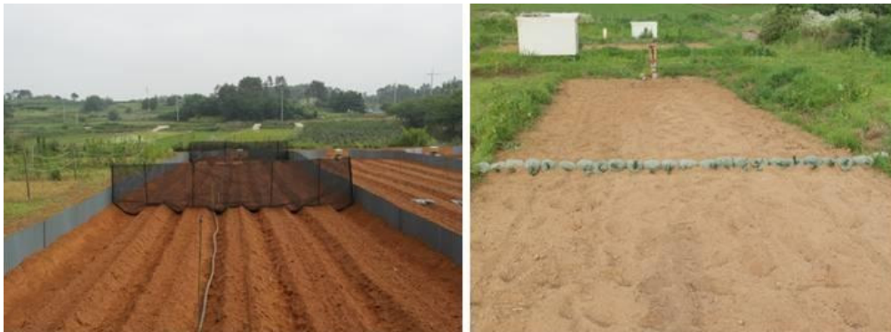
Fig. 4 Installed silt fence (left) and vegetated ridge (right)
