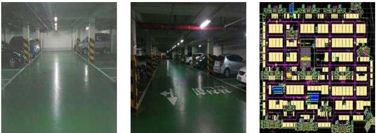
Fig. 1 Underground parking lot of ○○Building
