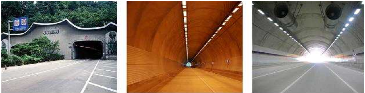
Fig. 3 Downtown area tunnel
