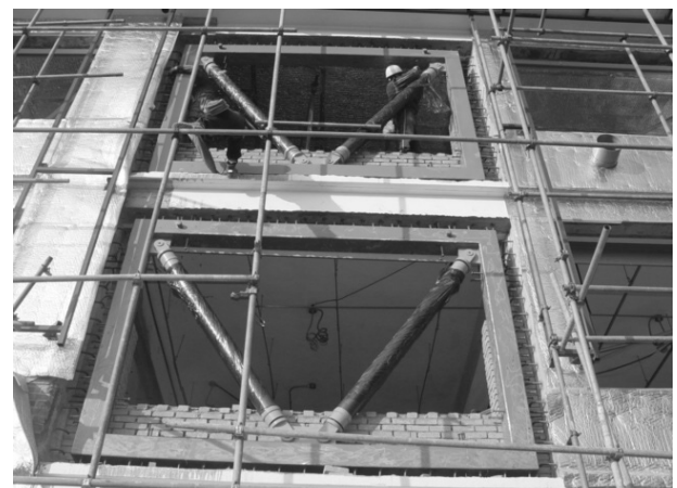
Fig. 1 Seismic retrofit example of RC school building
