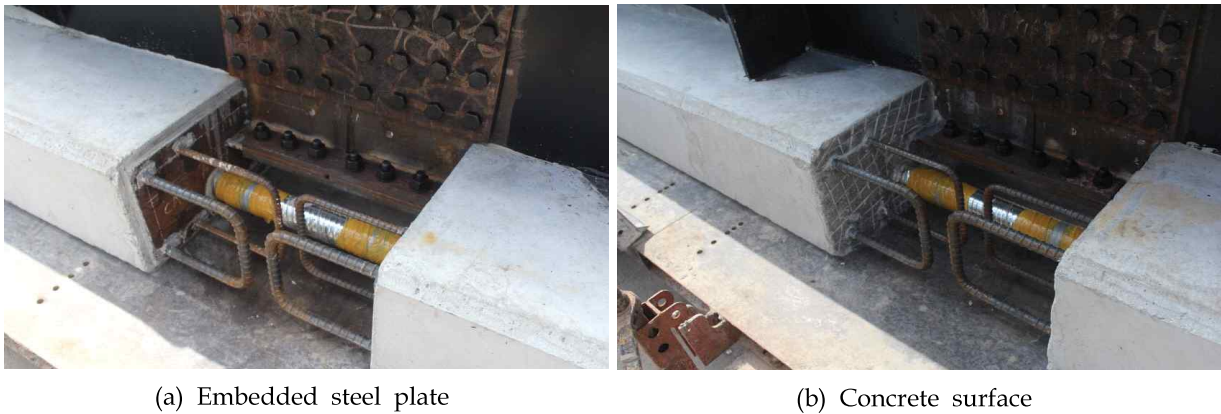
Fig. 4. Surface finish of the segments
