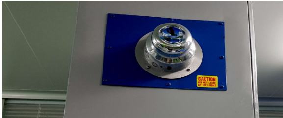
Fig. 2 REME System installed return duct.
