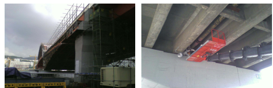
Fig. 2. Guidedwaves Inspection on River Crossing Pipeline.
