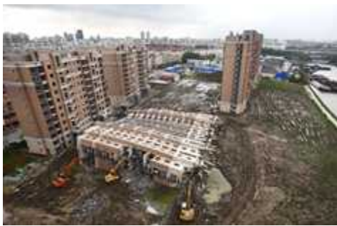
(a) Overall collapse for accumulated impertinently
