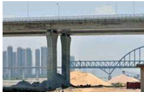
(b) Bulldozer near bridge piers
