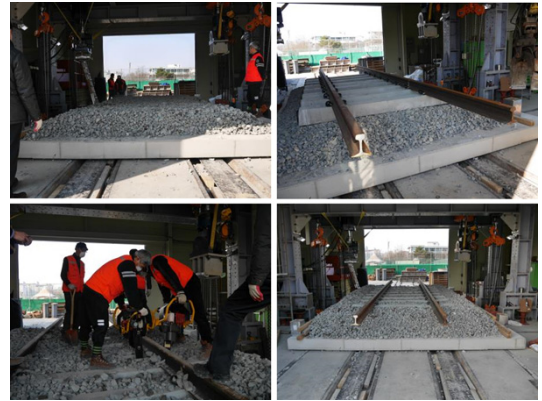
Fig. 7. Fabrication of track
