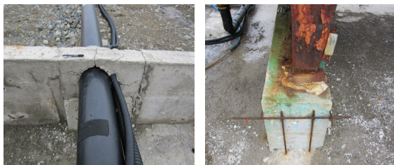
Fig. 2. Status of oil storage tank
