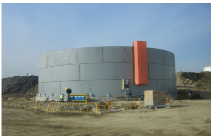
Fig. 1. Manual vertical welding of a huge oil storage tank
