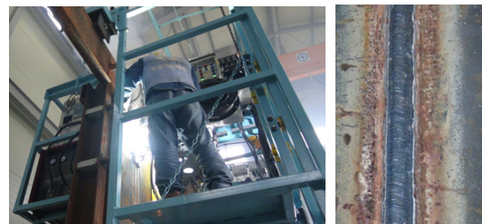
Fig. 15. Welding scene of the developed system and bead appearance
