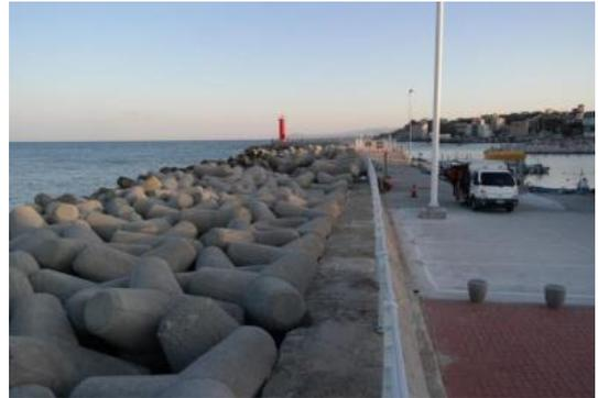
Fig. 1. Armor unit (Tetrapod) in a breakwater
