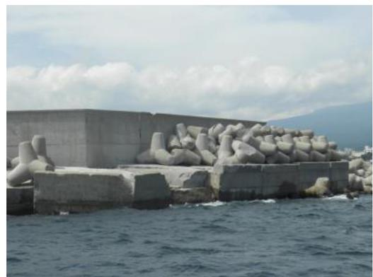
Fig. 2. Damage of breakwater in Seogwipo port, Jeju
